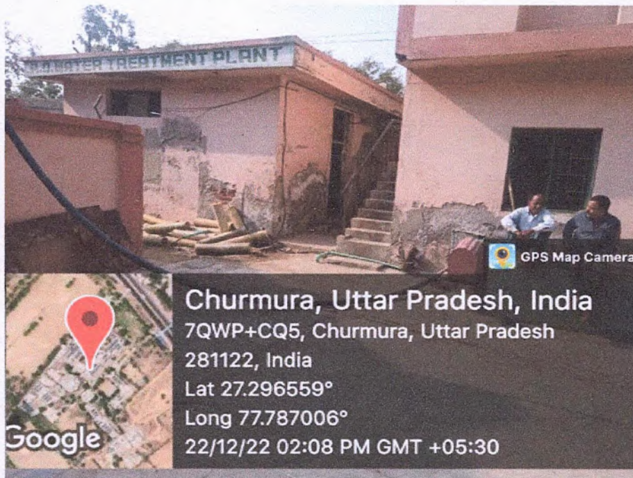
R.O. Treatment Plant, HCST Campus
