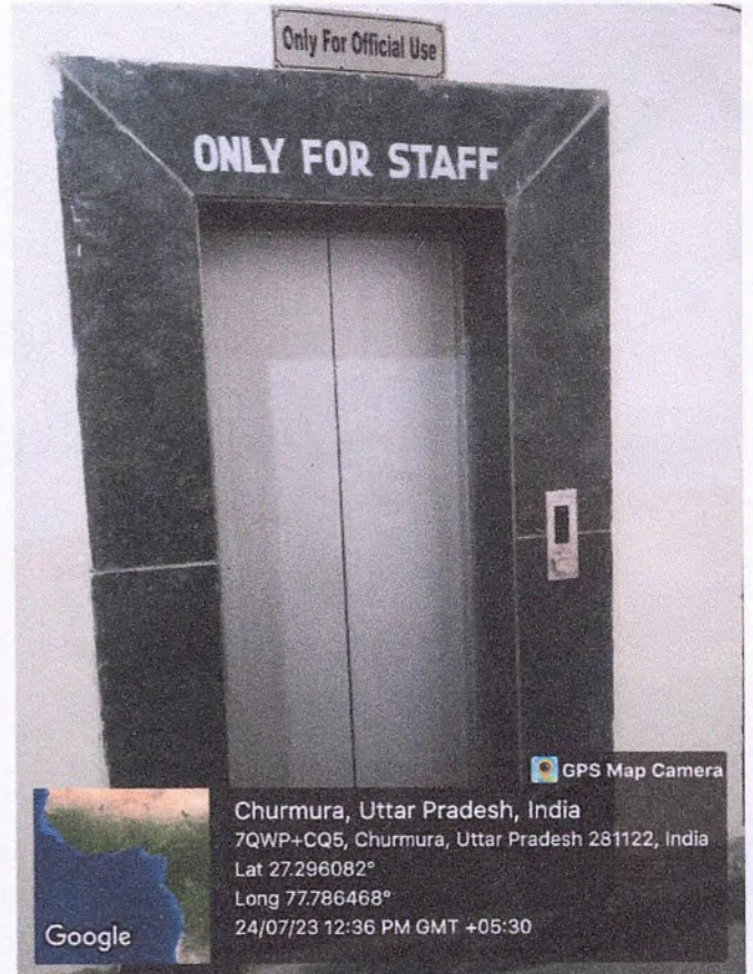
Lift Main Building
